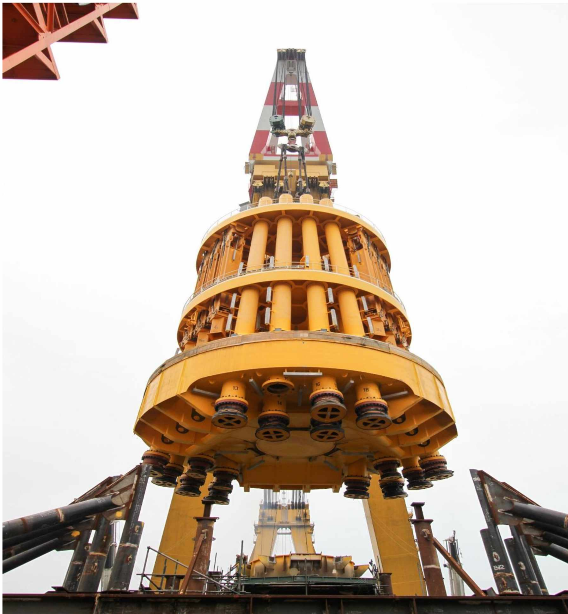
Kaombo Lifting South Turret
